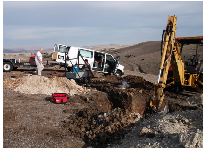
Figure 2.26.1. Installation of the seismic vault at TremorScope station TRAM.
